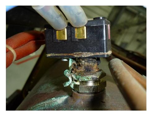
Figure 54 Corroded over-temperature switch (Image No. P1050563.jpg)
